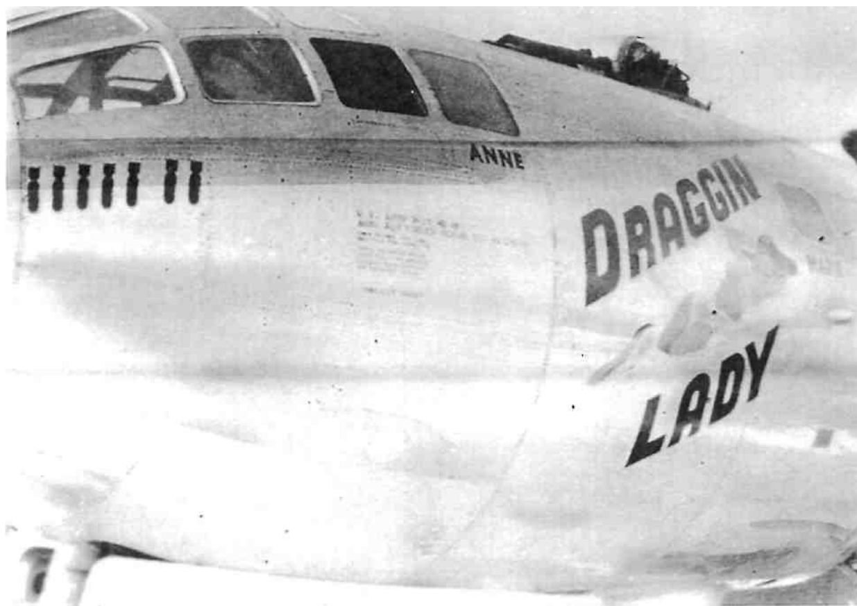
Another view of the nose art on "Draggin Lady" from a slightly different angle. Note the seven mission markings on the nose. Also, the dome covering the upper four gun turret has been removed, probably for maintenance on the guns. (Photograph from the Duane Blair Maples collection).
